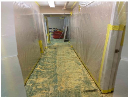
Central Ed. – Abatement contractor material removals in progress.
