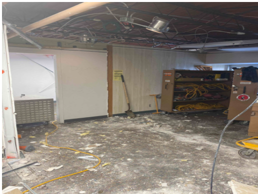
Central Ed. – Abatement contractor material removals in progress.
