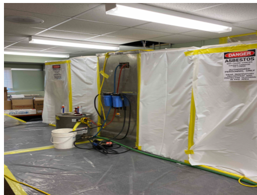
Central Ed. – Abatement contractor material removals in progress.
