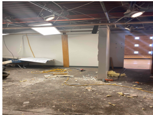
Central Ed. – Abatement contractor material removals in progress.
