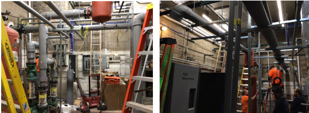
Central Ed. – Hydronic piping installation in the lower-level.
